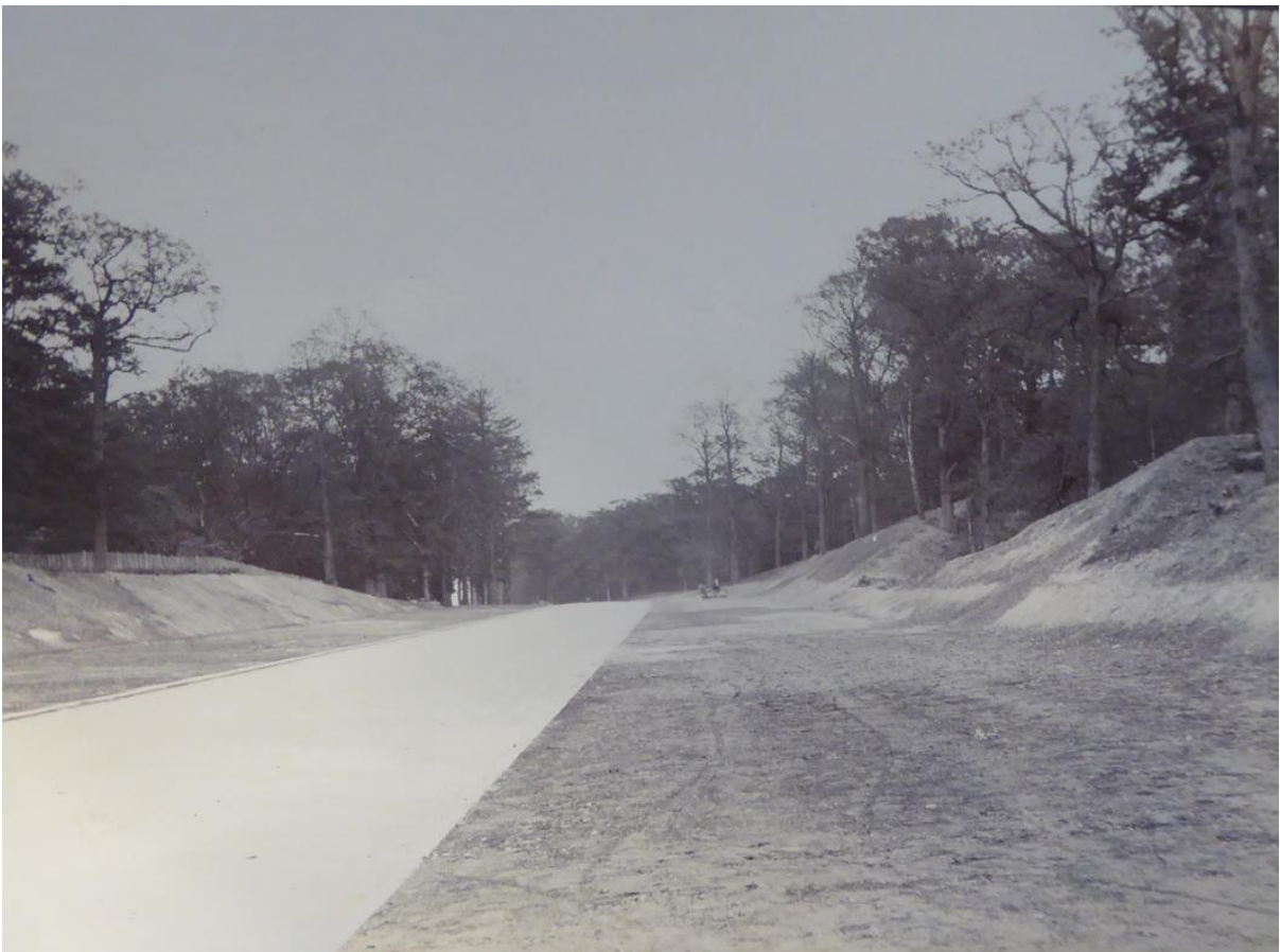
New road as built looking eastward from Thong Lane. Image © and reproduced by courtesy of The National Archives reference MT39 774 (dated 1924)
